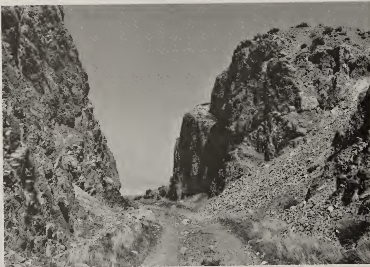
Figure 90: A large rock cut for the railroad grade in the Peplin Mountains. (BLM photo)
